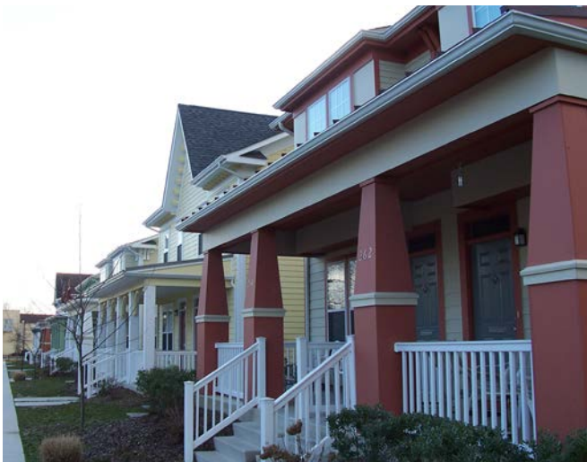
ComTec's Video Management System provided Bridgeton Commons with a state-of-the-art, cost-effective solution to its security and surveillance needs.
