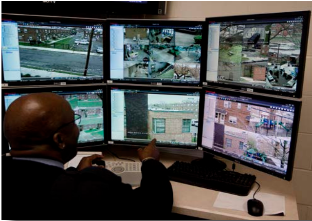
Video streams from throughout the city converge in one central command location at the Trenton Housing Authority.
